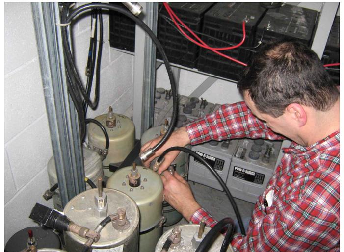
*Photo of Charles VE2RFI working on the VE2RWI repeater's multicoupler. A big thanks goes out to Charles VE2RFI, J-F VE2TBH, George VE2NGH, Leo VE2SI, Keith VE2MTL and Claude VE2YI for the good work.*
